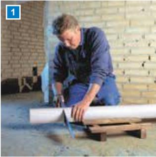
The pipe is cut at right angles with a fine-toothed (1-2 mm) saw or cutting device which is specially designed to cut plastic waste water pipes.
