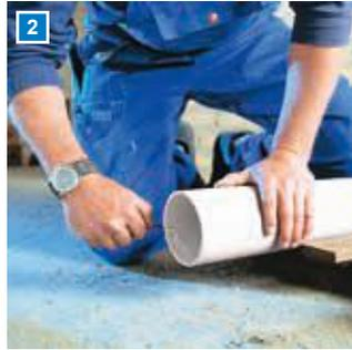
Then the end of the pipe is deburred on the inside and the outside. The ends of the pipes must not have any longitudinal scoring. The sealing groove and the sealing ring of the sleeve must be clean and free of any damage.
