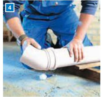
The pipe is then inserted into the sleeve, up to the insertion mark. The thermal expansion of the pipe must be taken into consideration when making all the junctions and connections.
